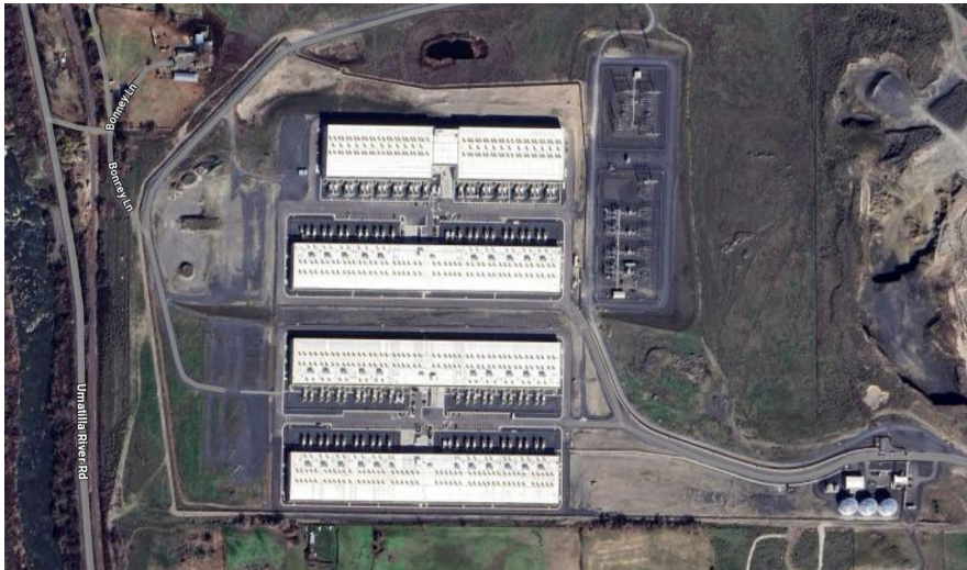
Amazon data center in Umatilla County, Oregon, 2025
