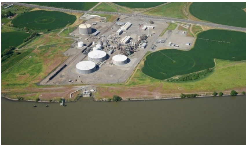
Agrium Fertilizer Facility in Finley. Photo Credit: Washington Department of Ecology, 2017
